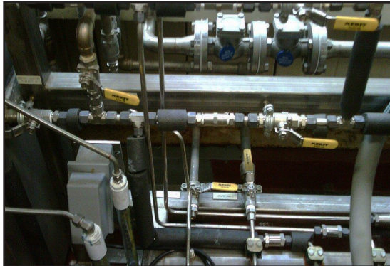
Power plants use a tremendous amount of compressed air, often an area for significant savings.
